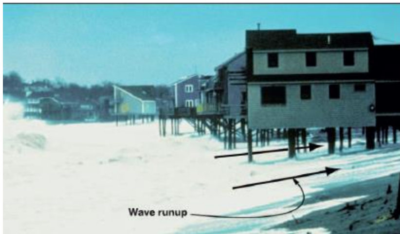
Figure 1.1. Wave runup beneath elevated buildings at Scituate, MA, during the December 1992 nor'easter storm. Source: Jim O'Connell, Coastal Construction Manual, fourth edition, FEMA P-55, Vol. I, August 2011.
